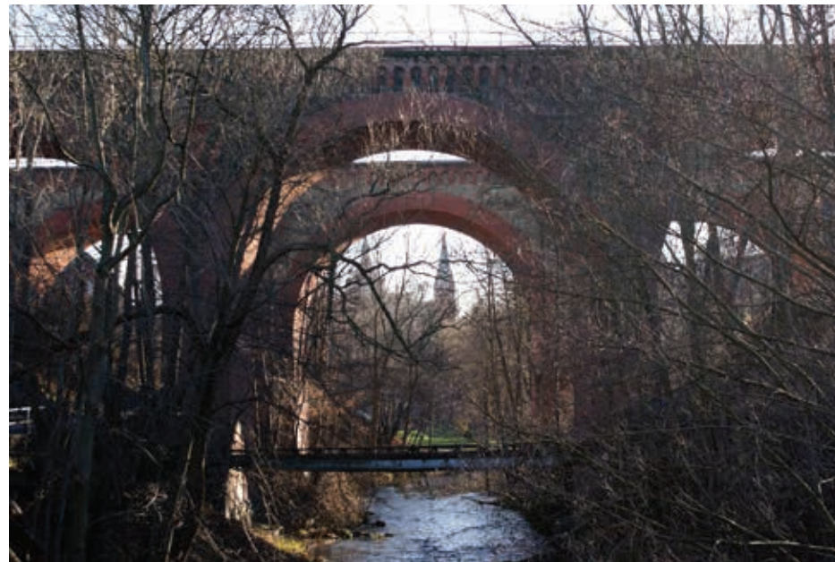
Mosty kolejowe w Olsztynie Railway bridges in Olsztyn
